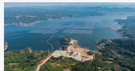
Cirata Floating PV Project
